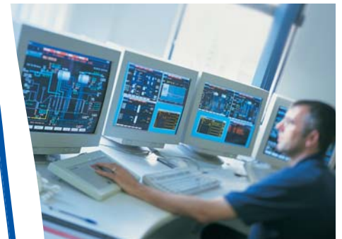
Critical applications requiring two independent electrical sources.
